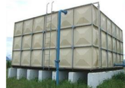
FRP WATER STORAGE TANK
